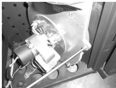
Figure 19 - a) Remove the screws; b) Remove extractor
