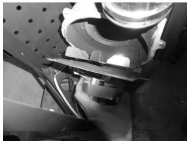
Figure 19 - a) Remove the screws; b) Remove extractor
